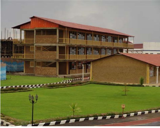
Example of building structure composed of earth bricks
